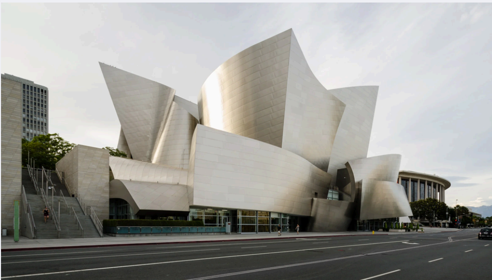
Gehry, Frank. Walt Disney Concert Hall. Los Angeles, USA.
